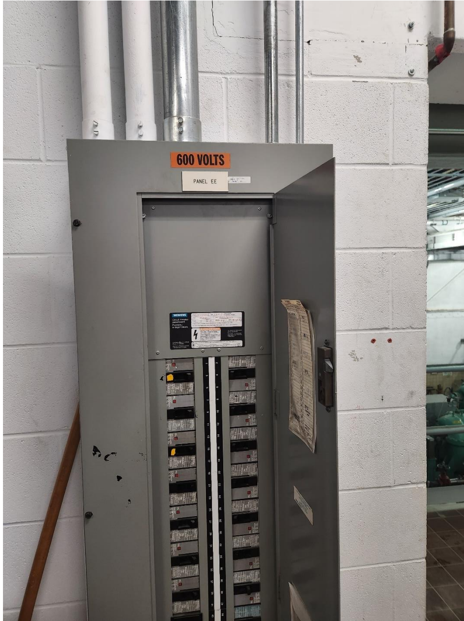
PHOTOGRAPH 62: Hurst Regional Pumping Station – Pumphouse Electrical Area – 600V Panel EE
