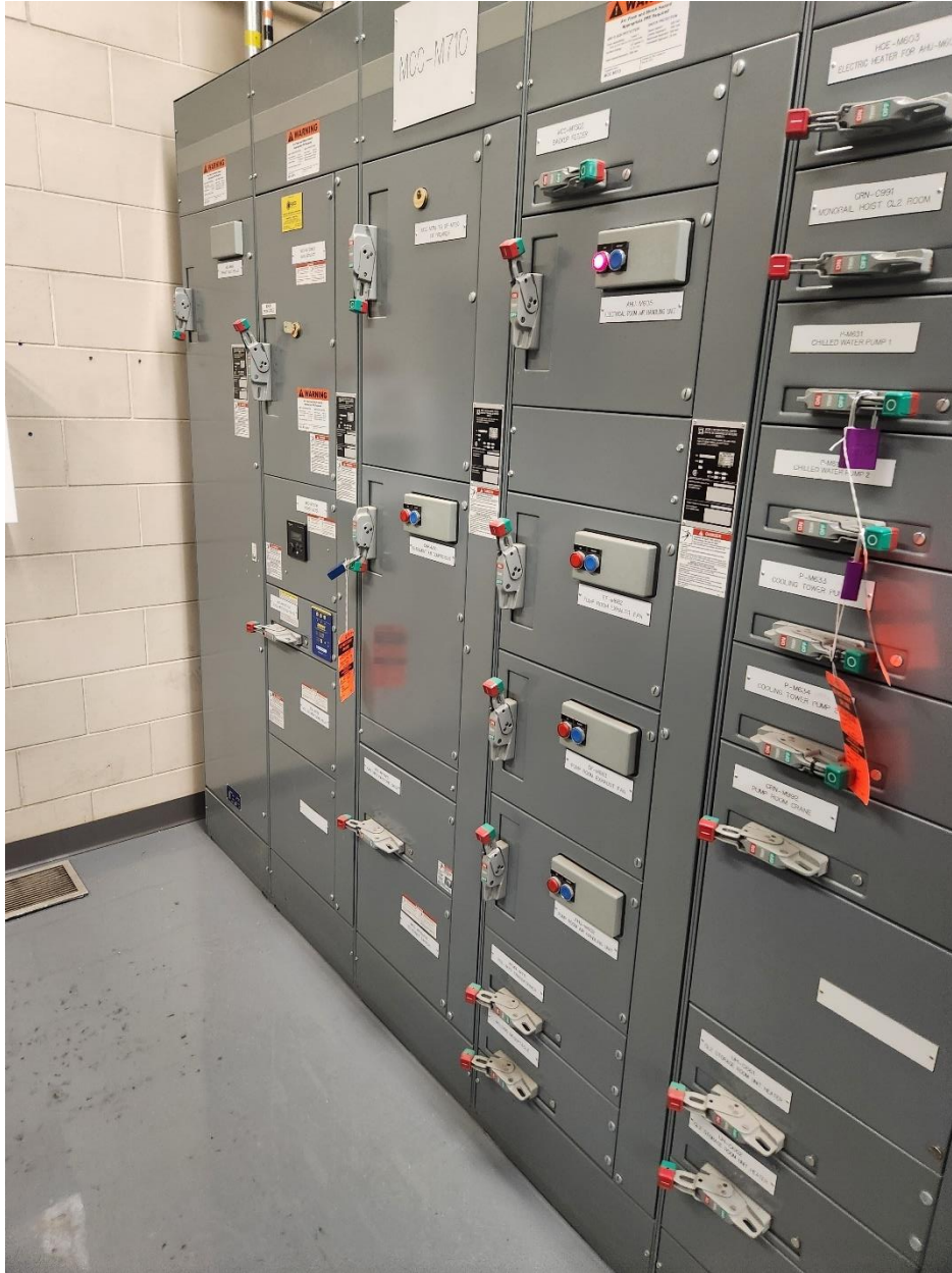
PHOTOGRAPH 39: MacLean Regional Pumping Station – Pumphouse Electrical Room - 600V Non-Essential MCC-M710
