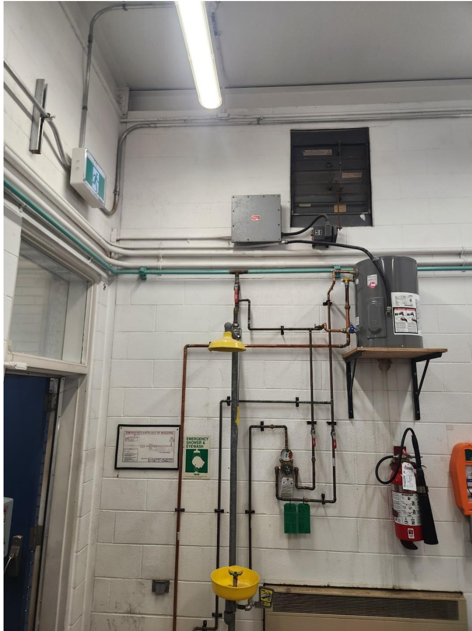
PHOTOGRAPH 2: McPhillips Regional Pumping Station – Chlorine Equipment Room East Wall – Existing Safety Shower System
