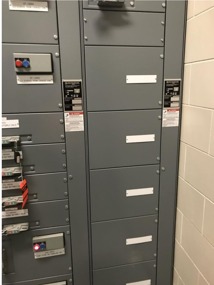
PHOTOGRAPH 41: MacLean Regional Pumping Station – Pumphouse Electrical Room - 600V Essential MCC-M730E
