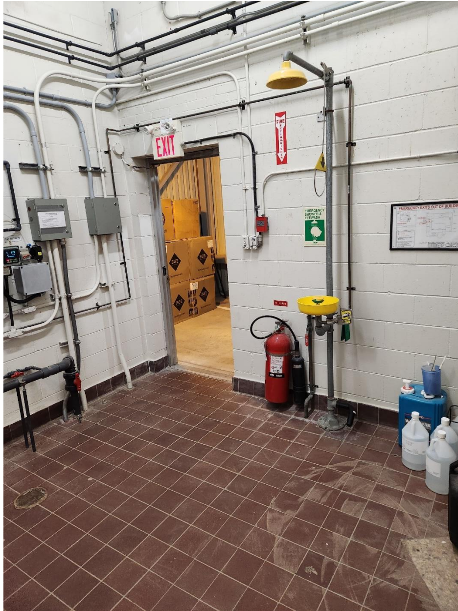
PHOTOGRAPH 44: Hurst Regional Pumping Station – Chlorine Equipment Room – Existing Safety Shower
