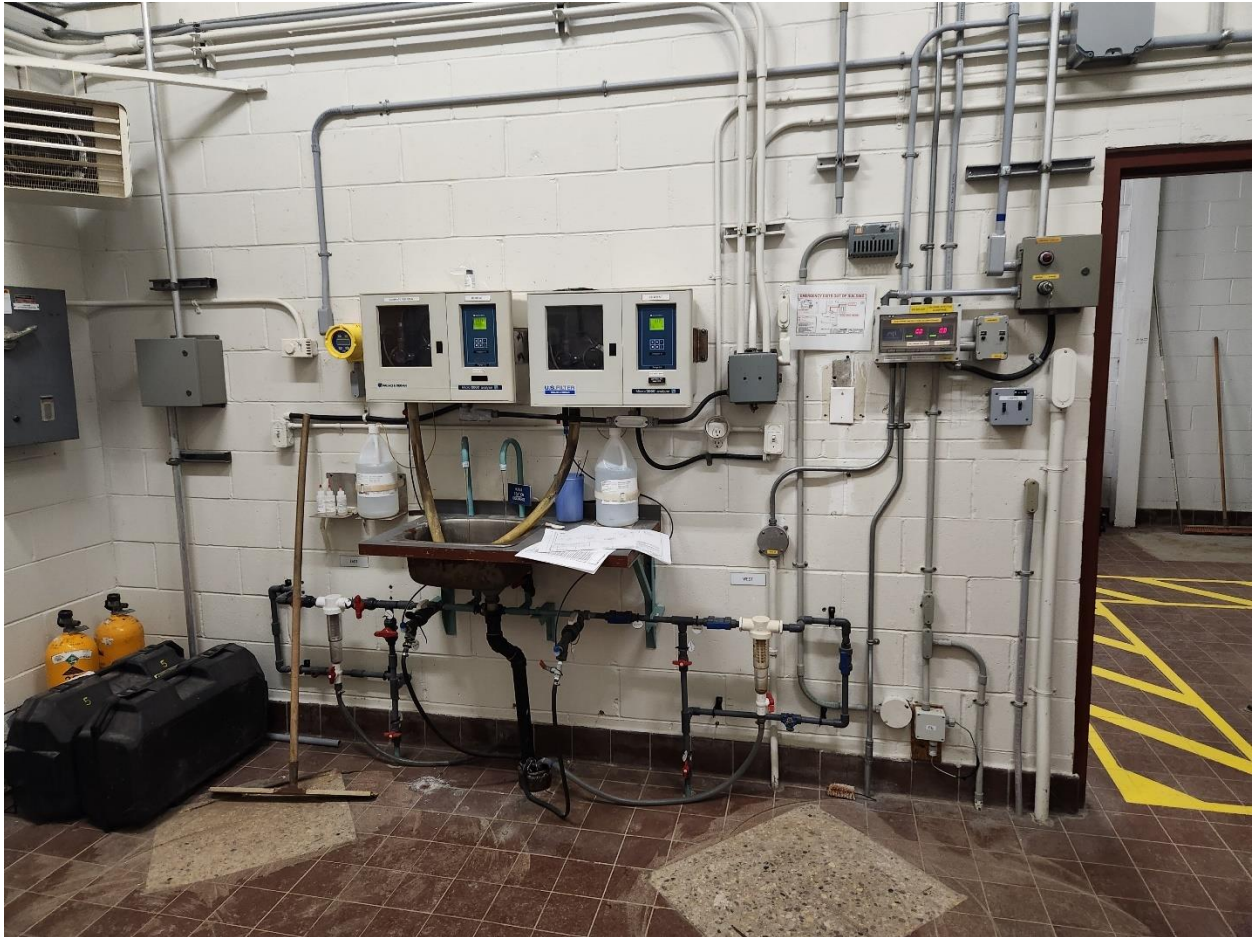
PHOTOGRAPH 43: Hurst Regional Pumping Station – Chlorine Equipment Room – South Wall – Existing Chlorine Detection System
