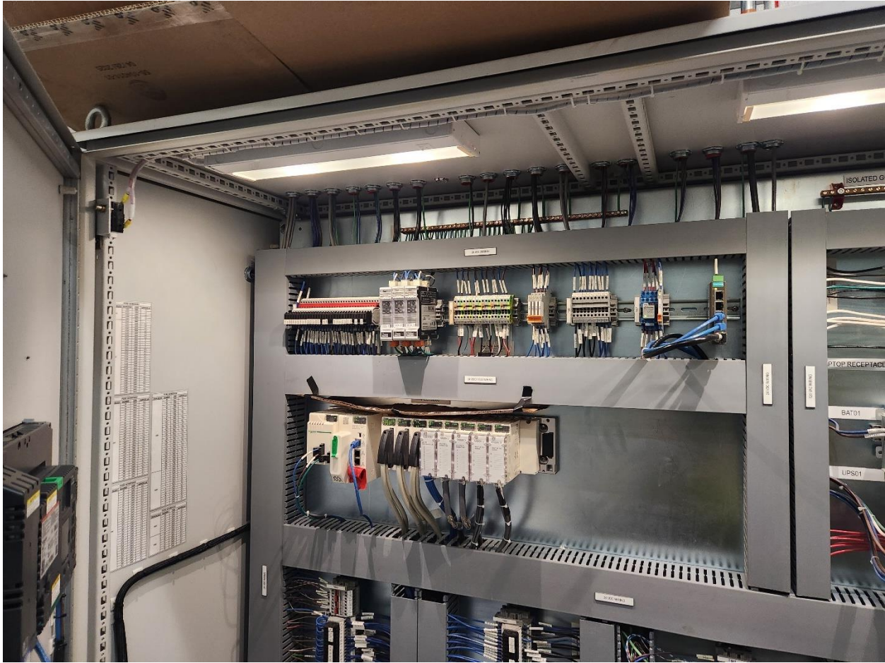
PHOTOGRAPH 21: McPhillips Regional Pumping Station – Pumphouse Mechanical Room – HVAC PLC Panel CP-M826 – Interior
