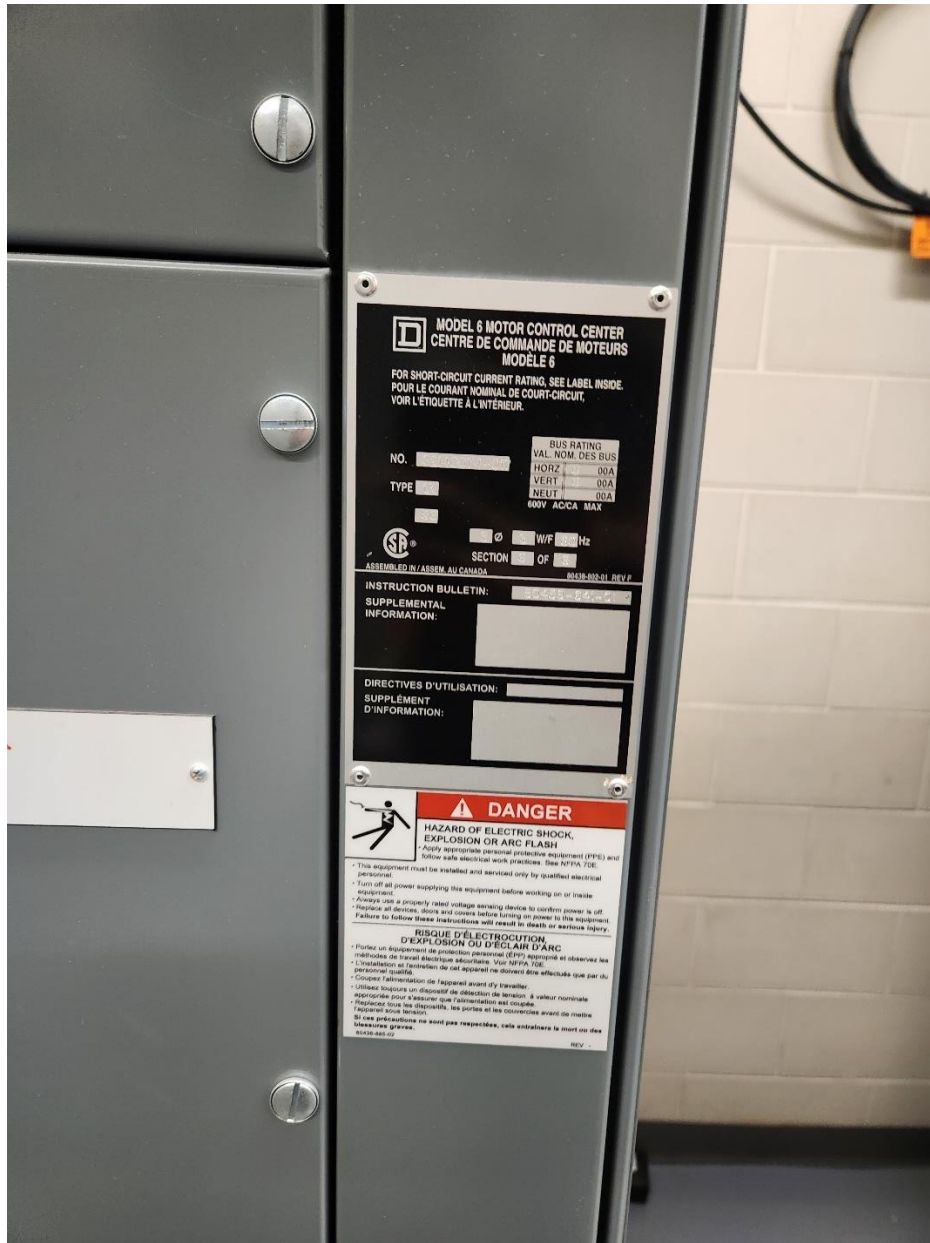
PHOTOGRAPH 40: MacLean Regional Pumping Station – Pumphouse Electrical Room - 600V Non-Essential MCC-M710 Nameplate
