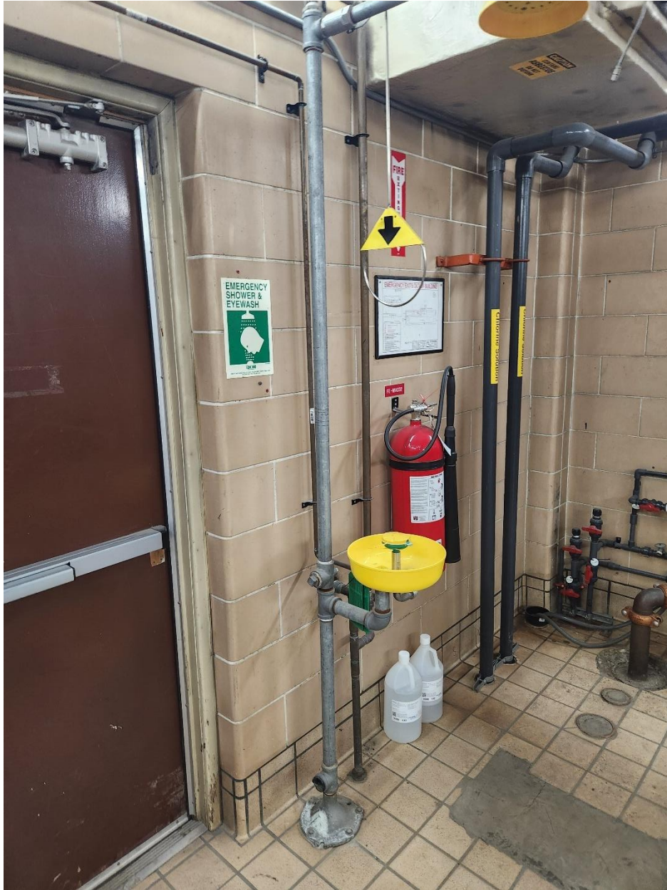
PHOTOGRAPH 24: MacLean Regional Pumping Station – Chlorine Equipment Room – Existing Safety Shower.
